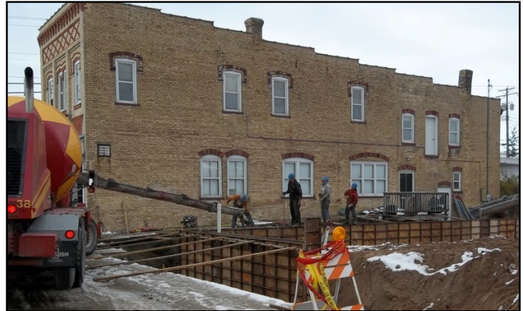
Workers from Schuh Construction pour the concrete foundation. You can follow the progress of the new building on the SCHS Facebook page.
