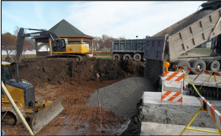
Prior to pouring the concrete footings and floor, the soil was excavated to a depth of ten feet and filled with crushed rock and sand. This was then compacted to form a solid base.
